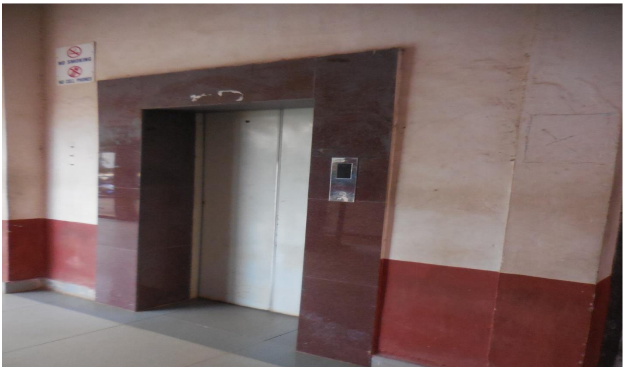
Lift Near Office
