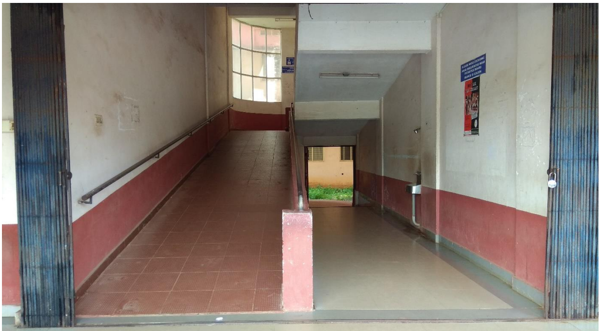
Ramp with guiderail
